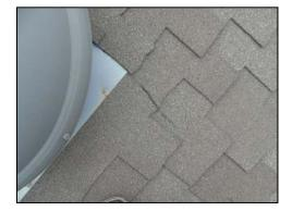
Defect Code:23Quantity:1Priority:MonitorDescription:Physical damage to membrane including cuts, holes, tears, scrapes, scuffs, or abrasions.
