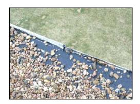
Defect Code:70Quantity:RandomPriority:First YearDescription:Open joint in metal flashing.
