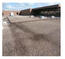
One (1) core sample was taken on the main roof area. The deck is a factory primed steel decking. The insulation consists of one (1) layer of 1.5" polyisocyanurate insulation board and one (1) layer of .5" wood fiber cover board. The membrane is a multiply BUR with a gravel surface.
