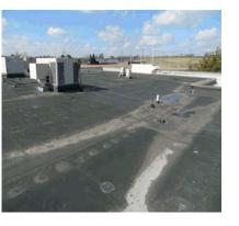
One (1) core cut revealed a steel decking and one (1) layer of 5/8" gypsum board. The insulation consists of two (2) layers of 4" air-expanded polystyrene and a .5" layer of wood fiber cover board. The membrane is a fully-adhered, .060 mil Firestone EPDM. The wood fiber board was partially deteriorated at the core cut location. The depth of the roof system was checked at an additional location and the insulation does not appear to a tapered system.
