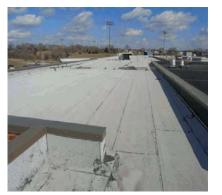
One (1) core cut revealed a steel decking. There are two (2) layers of 1.75" polyisocyanurate board and a .25" layer of Dens-Deck cover board. The membrane is a two (2) ply SBS modified bitumen with a granulated surfacing.
